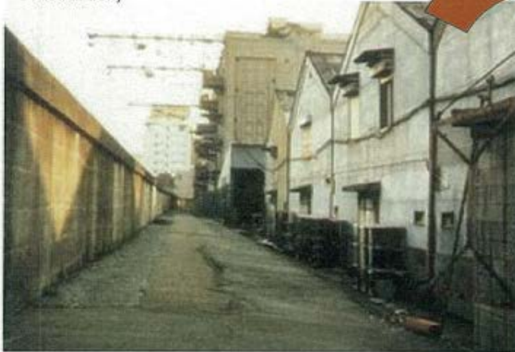
▼Sumida River, Shinkawa/Hakozaki Districts (before construction)
